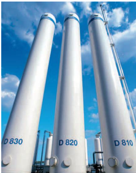
Figure B-25: Pressure vessels applied for industrial hydrogen storage at 50 to 70 bar (left, (Belloni 2003)) and gasometer formerly used for hydrogen-rich gas storage (right, www.gasometer.de ).
